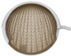
Timber lattice domes were built from double-curved laminated timber beams.
