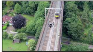
High-res imagery captured even during traffic hours
