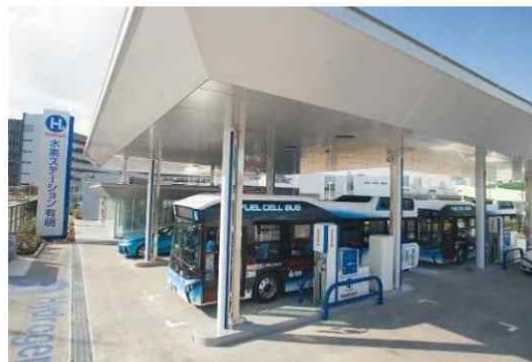
Tokyo-Ariake Hydrogen Station (Source: Iwatani's website)
