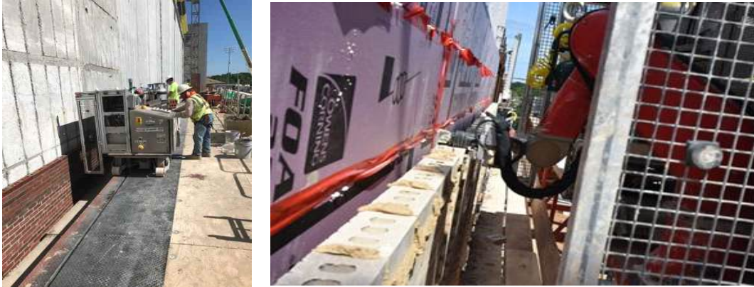
[그림 19] SAM(Semi-Automated Mason) (출처:Construction Robotics)
