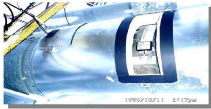
M2 sensors Fitted on Pipelines prior to insulation being reinstated
