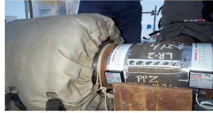
M2 sensors Fitted on Pipelines prior to insulation being reinstated
