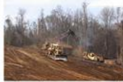
Typical site is mass cleared
