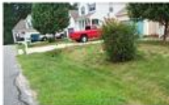
Vegetated open channel
