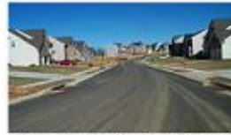
Typical excessively wide road
