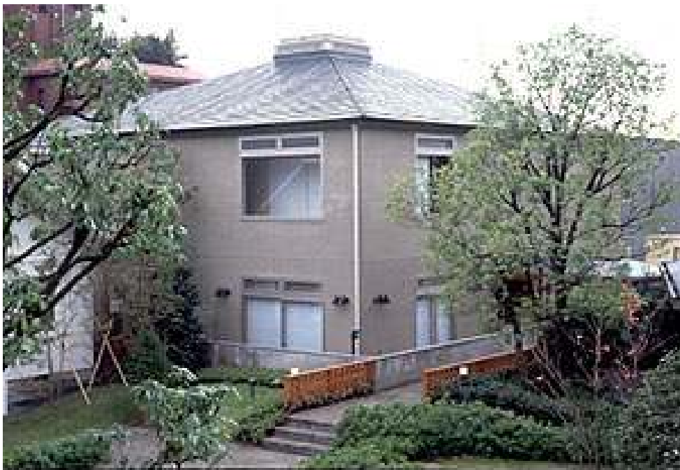
Front of the TRON Intelligent House
