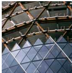
Construction Logistics / PM
