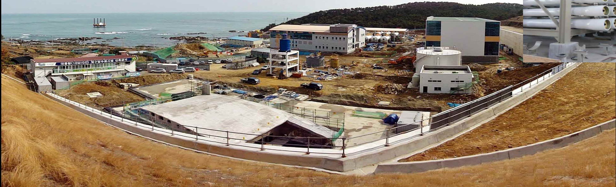
SeaHERO RO plant in Busan, Korea
