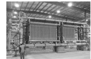
(b) Membrane ultra-filtration unit
