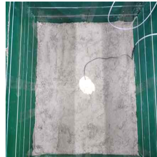
(b) Earth pressure gauge installation
