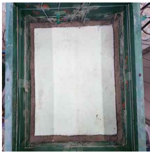
(c) Concrete mat installation
