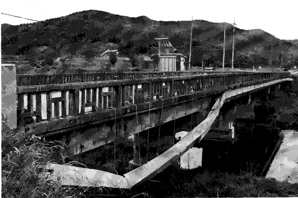
(b) side view of Ssanggye bridge
