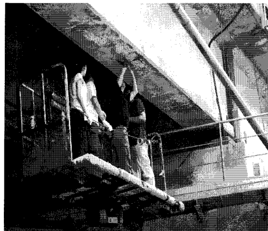
Fig. 4-46 Sensor attaching work
