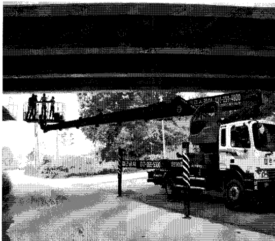
Fig. 4-45 Sensor attaching work
