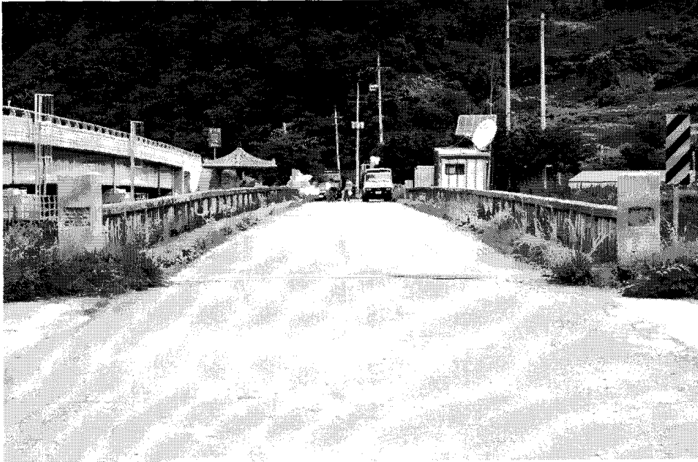
(a) front view of Ssanggye bridge
