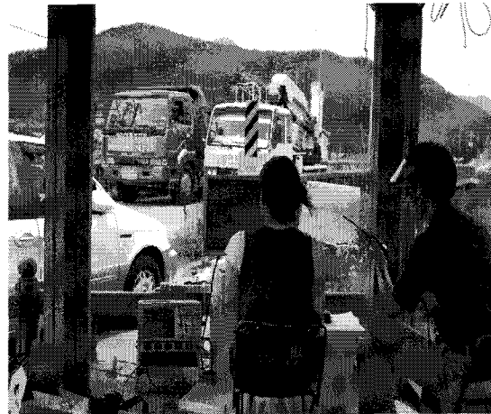
Fig. 4-14 AE measurement at site
