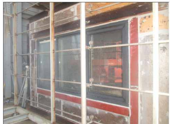
나) Water Spray Rack
