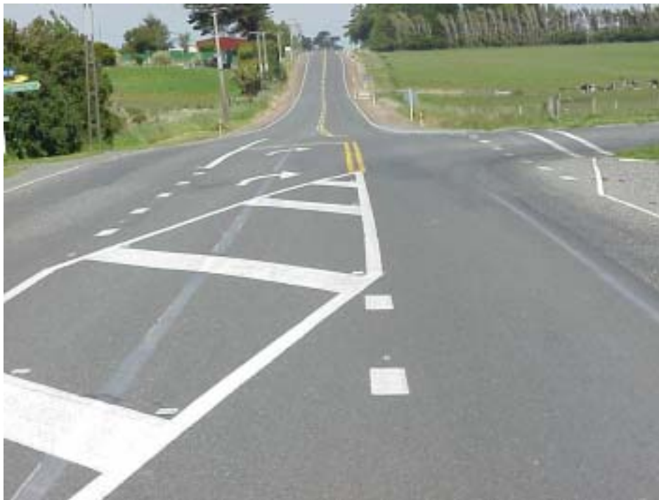
Unsafe delineation from 'blacked out' unwanted centre and edge lines. Glass bead was clearly evident on the blacked out markings. Tests showed these lines had higher reflectivity than the new white lines and would therefore be more visible at night (reflectivity readings of 111 and 64 on the blacked out lines, compared with 58 to 80 on the new white lines).
