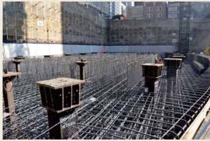
Rebar Placement Mat Foundation Wilshire Grand
