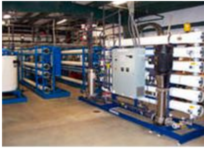
(a) Membrane ultra-filtration unit
