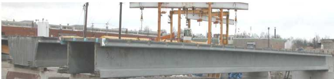
(c) Fedral Highway Administration Bridge, USA (2005)
