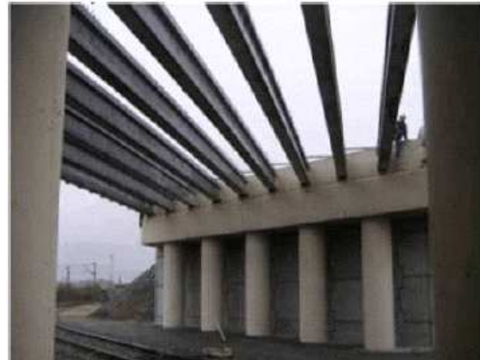
(b) Saint Pierre La Cour Bridge, France (2005)
