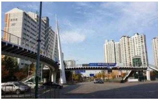
(a) A Bridge Panorama
