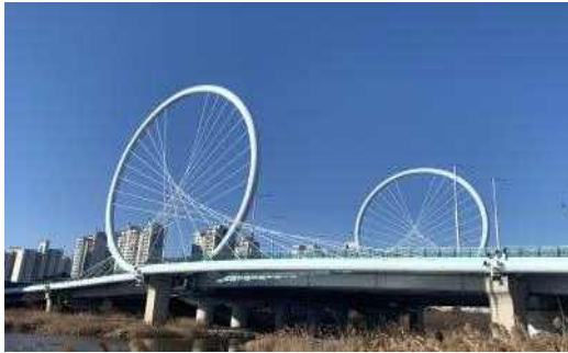
(b) B Bridge Panorama
