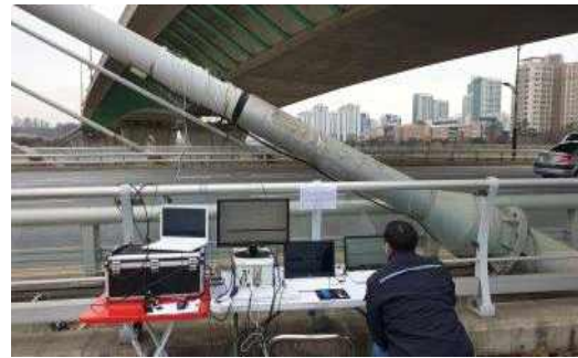
(c) C Bridge Cable Tension Measurement
