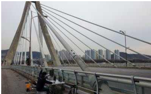
(c) C Bridge Panorama
