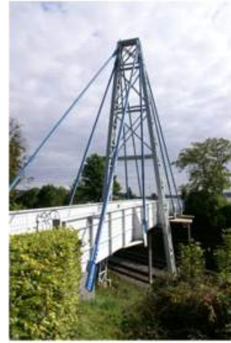
(b) Kolding Footbridge in Denmark
