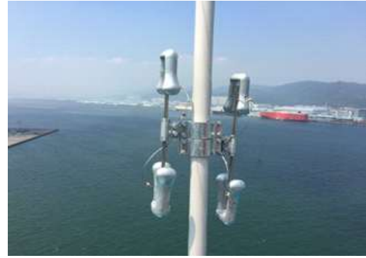
<울산대교 Stockbridge Damper (2015), [출처: TE Solution]>
