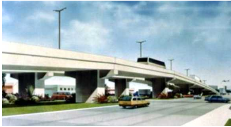
<Baldorioty de Castro Avenue Bridge, San Juan, Puerto Rico>
