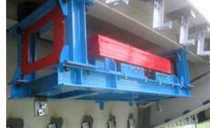
<울산대교 Stockbridge Damper (2015), [출처: TE Solution]>
