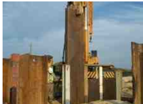
(f) Steel Plate 삽입
