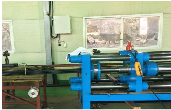
(b) TIE-CABLE 제작공장(압착)
