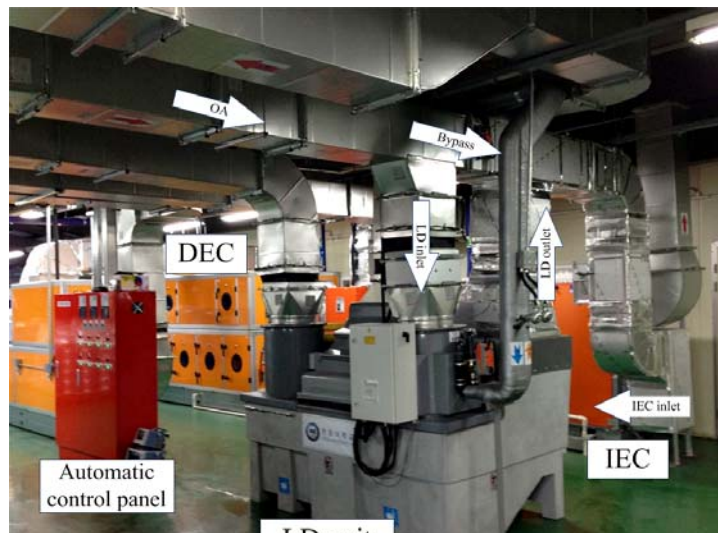
(a) 제습 증발냉각시스템 Proof-of-concept 실험
