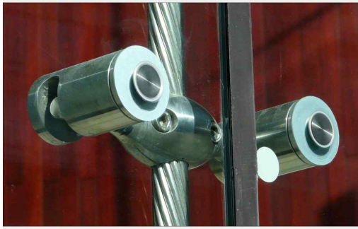
[그림 4.2] Cable Mullion System : Juilliard Alice Tully Hall, Entry Wall, New York
