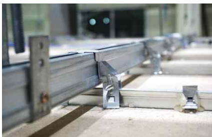
T-Bar &amp; Carring channel 고정부
