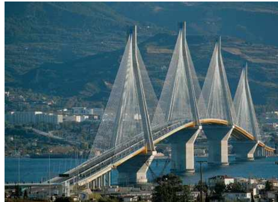
(b) Rion-Antirion Bridge
