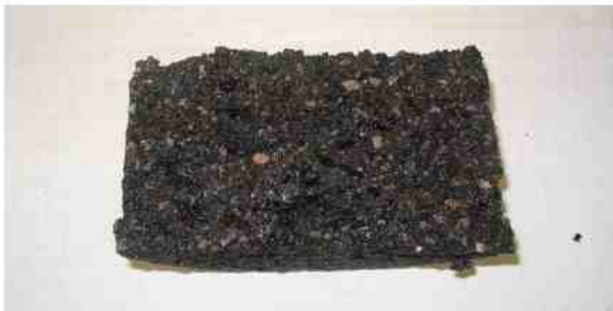
Figure 15. Example of Adhesive Stripping Failure – Granite
