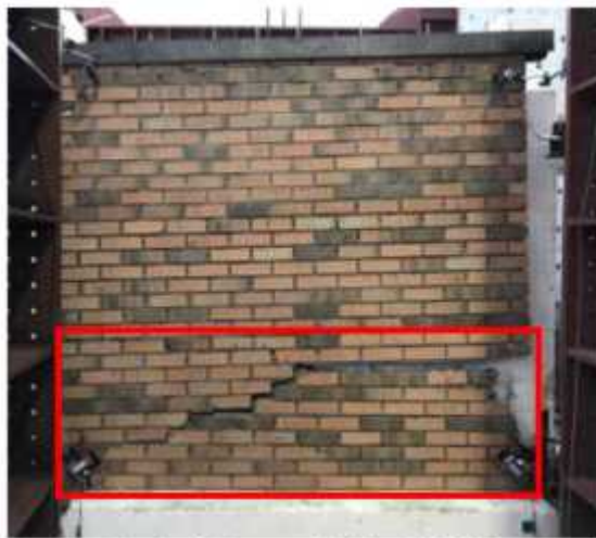
(a) Crack Pattern of EML-S600-L3-I
